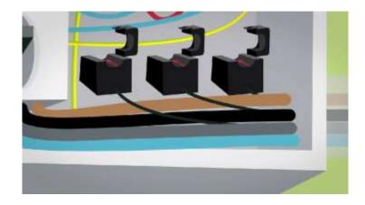
5. Plug the ends of the power clamp cables into input 1, 2 and 3 of the Smappee monitor
