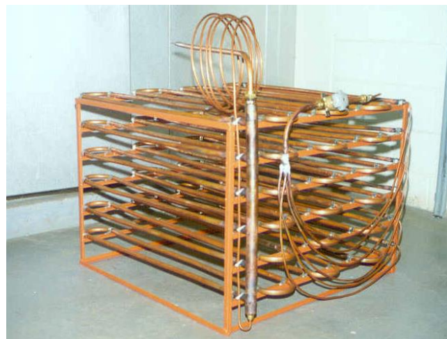
FIGURE 2. Evaporator built to the ice bank.
